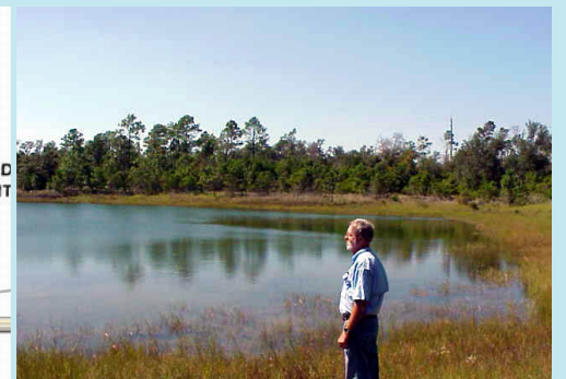
Inspecting a vegetated retention pond ( www.dep.state.fl.us )
