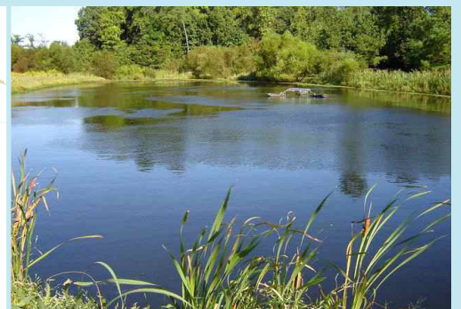
A vegetated retention pond ( www.solarbee.com/stormwater )
