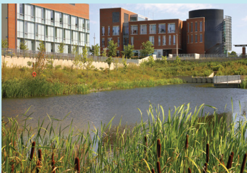
A commercial vegetated retention pond ( www.architectmagazine.com )
