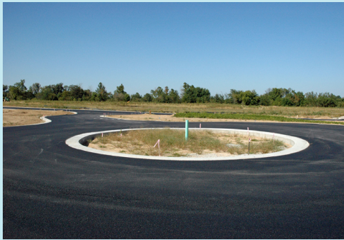
A recessed island during construction in Wood River, Illinois (William Freeman)
