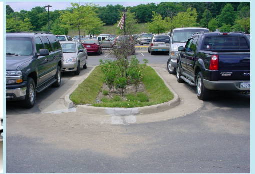
A retrofitted recessed parking island with curb cut (co.stafford.va.us)
